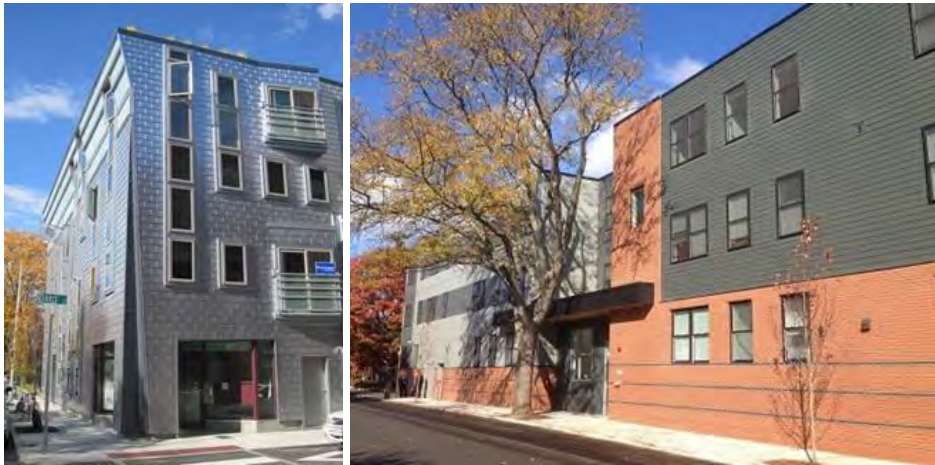
Figure 14 – Examples of newer multifamily buildings in The Port (credit: City of Cambridge)
