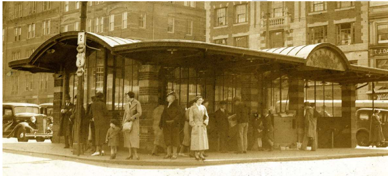
Kiosk, ca. 1938, functioning as headhouse (Boston Elevated Railway Collection, Cambridge Historical Commission)
