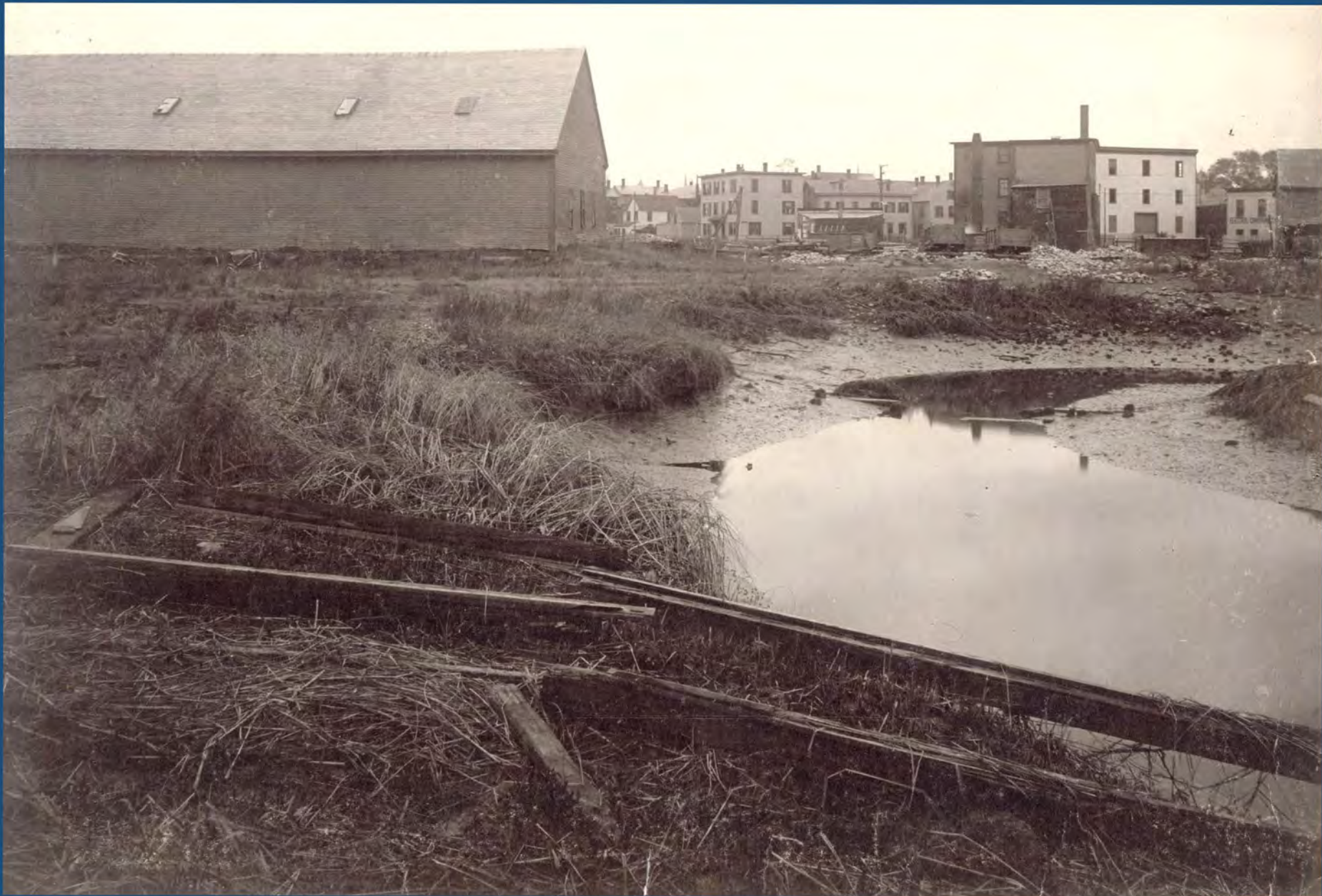
Natural outlet of the millpond creek, ca. 1895
