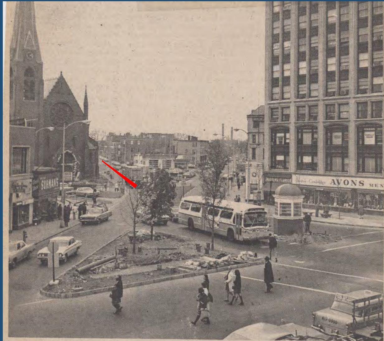
TREES IN CENTRAL SQUARE: - Pedestrians stare in wonderment at trees planted in heart of Central square as part of beautification program financed by city and federal funds. Like New York City, Cambridge will soon have its own "Central Park." Three maples and foundations for benches are shown in triangular plot, left foreground. At extreme right, sidewalk has been widened, trees have been planted and benches installed for weary shoppers. Traffic tower will eventually be removed. City's new "Mini Park" is conversation piece for miles around. (Photo by Ed Pacheco)
