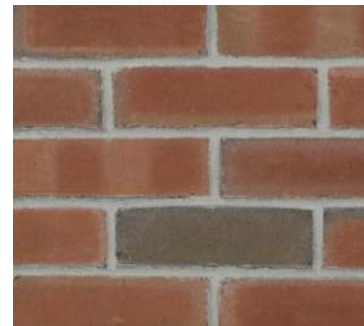
3 REBUILT BRICK WALL @ GREEN ST
