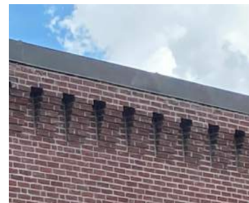
Photo of existing cornice to be rebuilt
