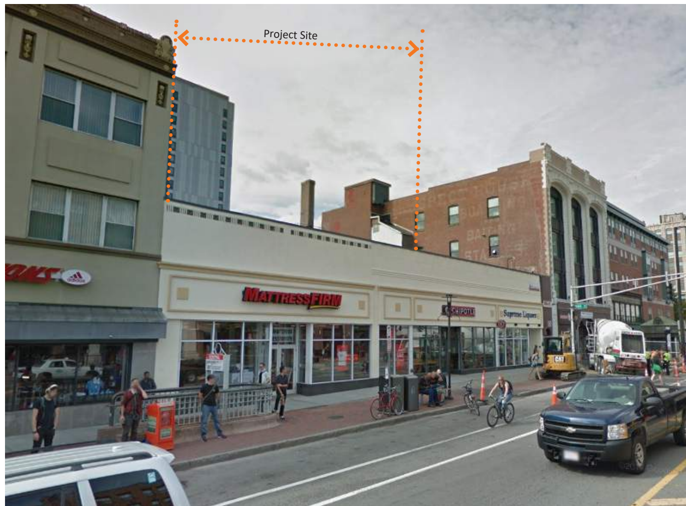
2. EXISTING MASS AVE. NORTH EAST VIEW
