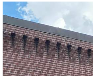
Photo of existing cornice to be rebuilt
