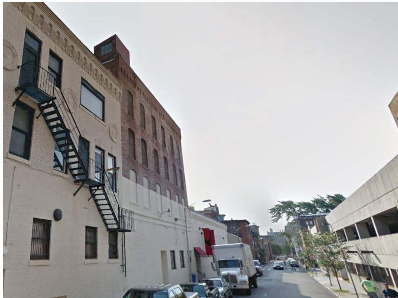
2. EXISTING GREEN ST. SOUTH WEST VIEW
