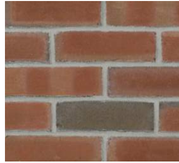
1 REBUILT BRICK WALL @ GREEN ST
