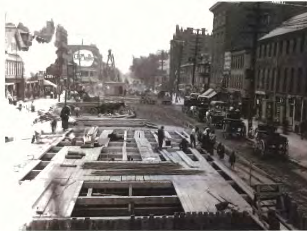
VIEW DOWN MASS AVE - C. 1910
