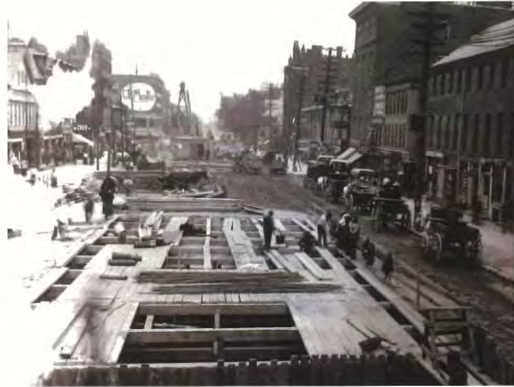
VIEW DOWN MASS AVE - C. 1910
