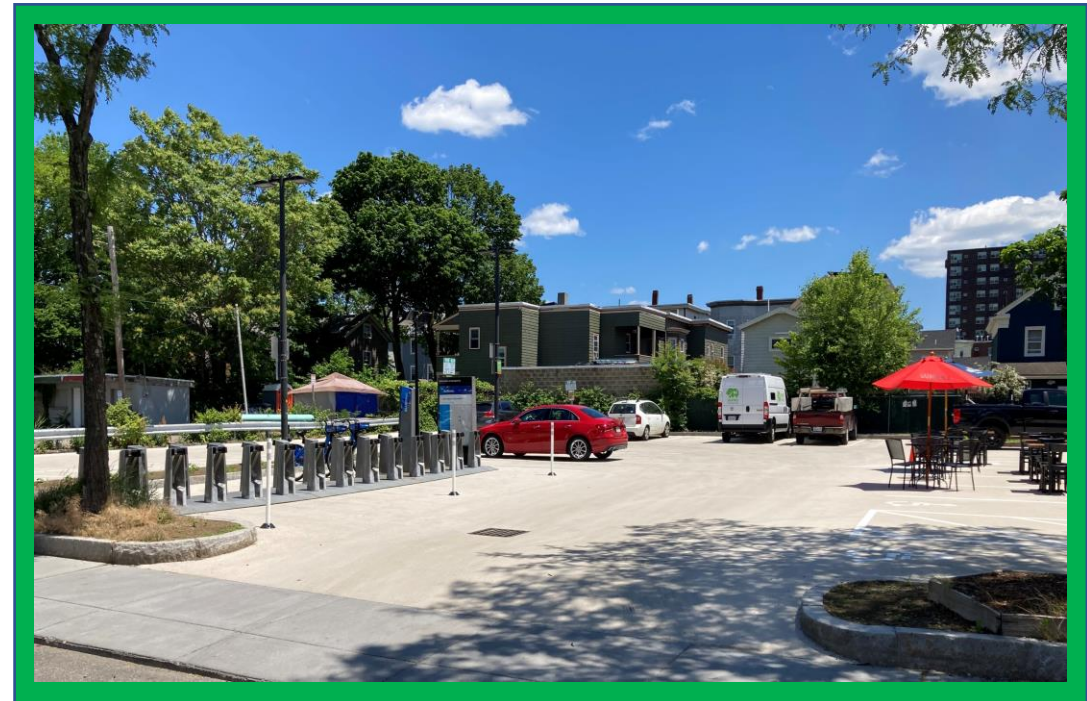
Springfield Street High Solar Reflectance Coating
