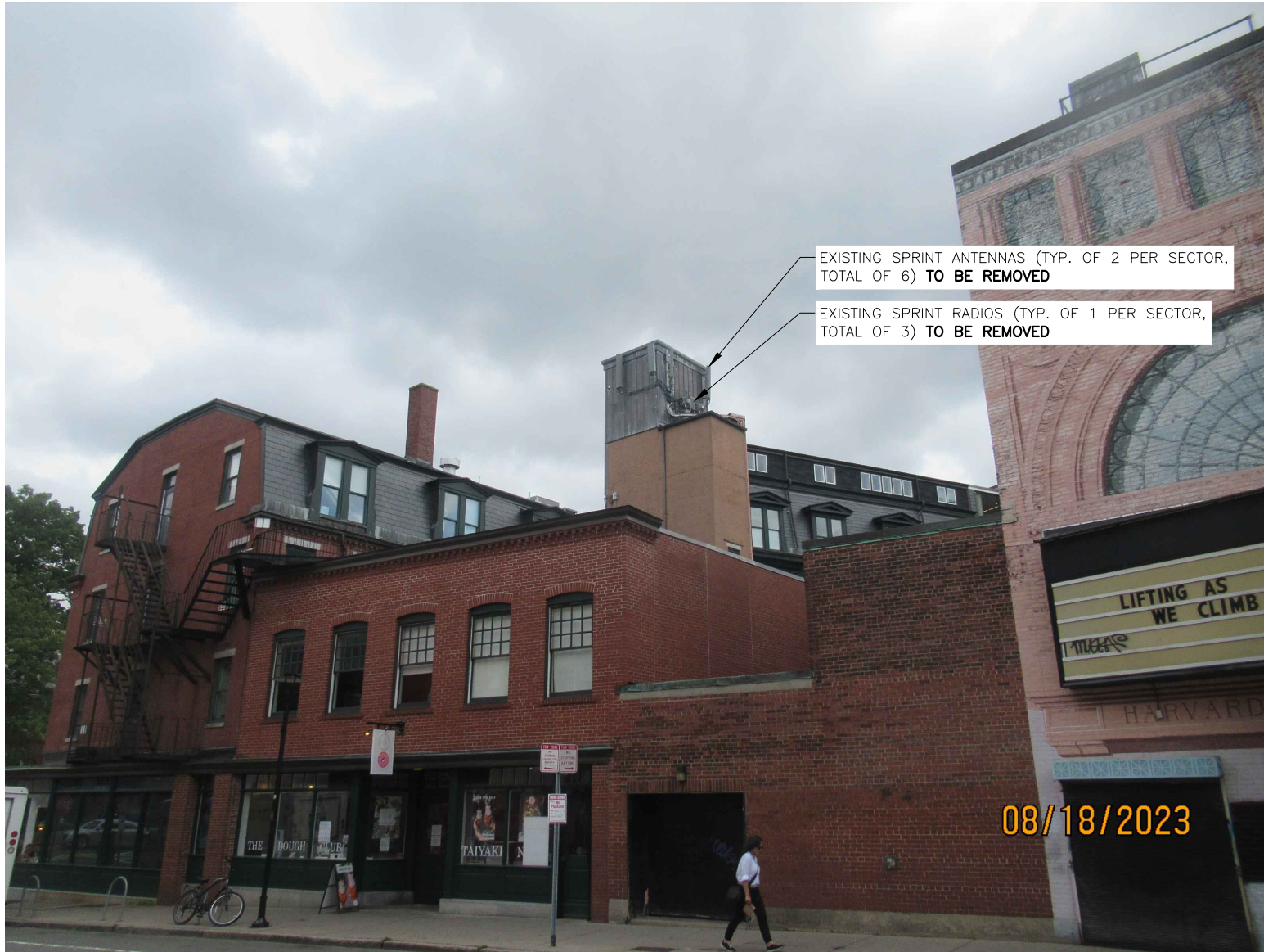
VIEW SOUTHEAST FROM CHURCH ST
