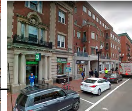
Existing metalwork details on Massachusetts Avenue
