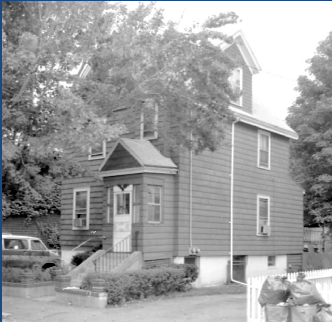
19 Cottage Park Avenue, CHC Photo, 1982.
