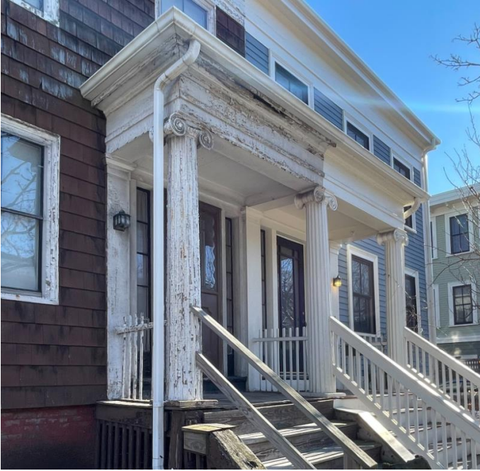
Portico detail at façade of 194-196 Prospect Street.
