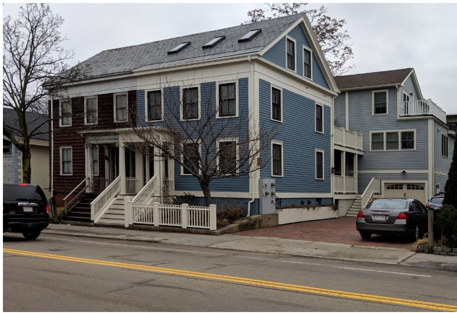
194-196 Prospect Street as photographed in 2021.. 194R Prospect Street is seen at right.
