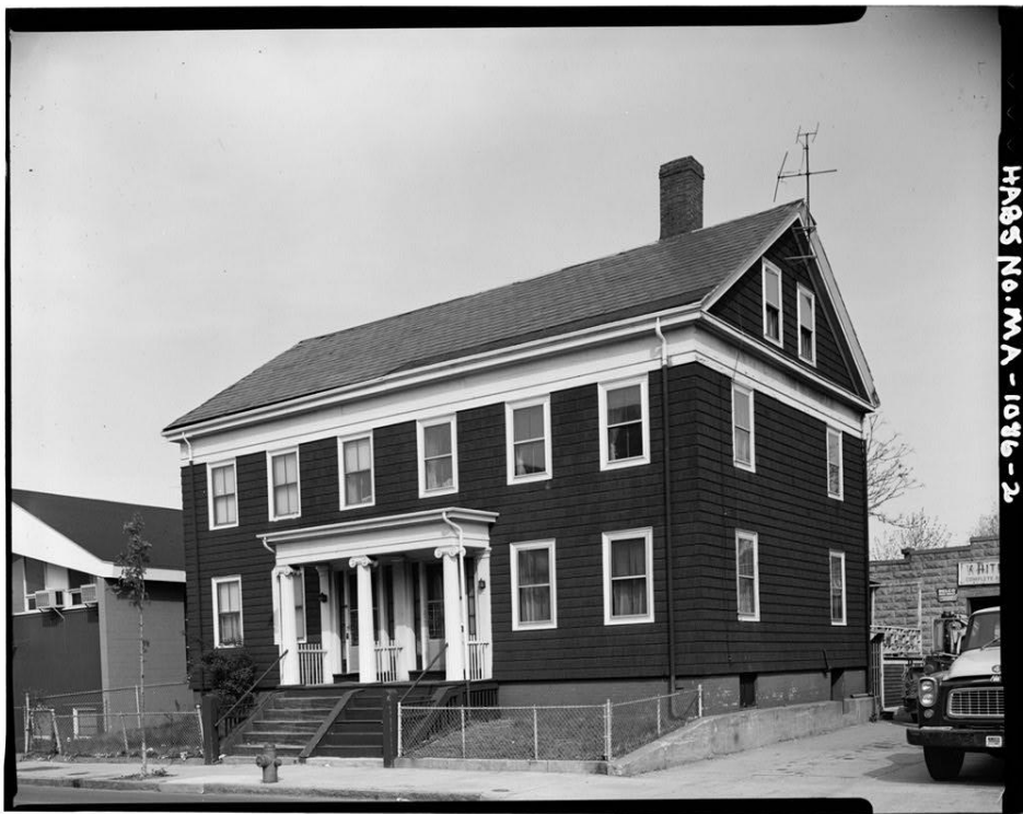
194-196 Prospect Street, c.1987. Historic American Buildings Survey photograph.
