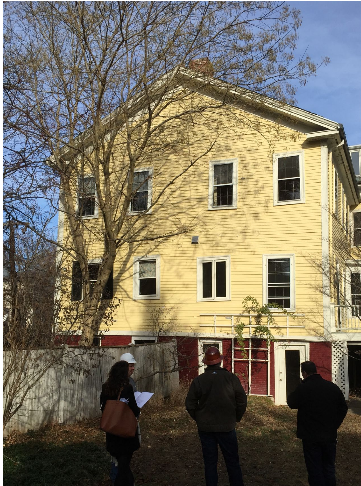
EXISTING SOUTH FACADE VIEW
