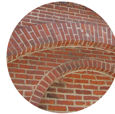
MASONRY Historic Brick
