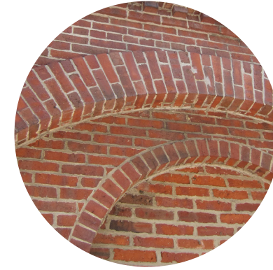
MASONRY Historic Brick
