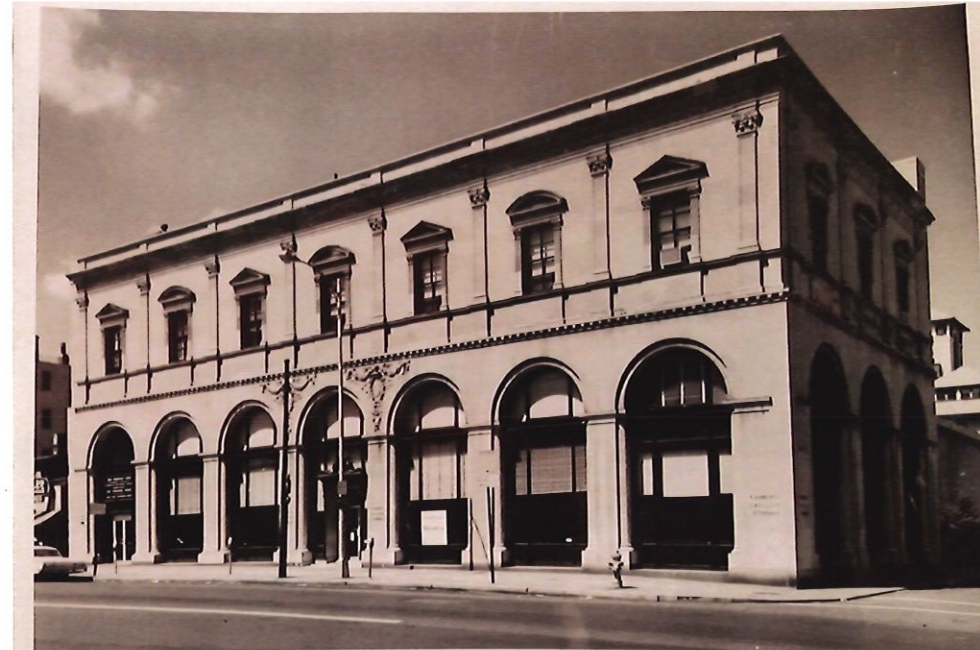
View from Massachusetts Ave
