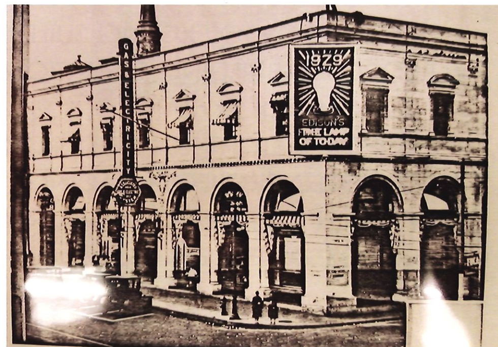
View from Massachusetts Ave
