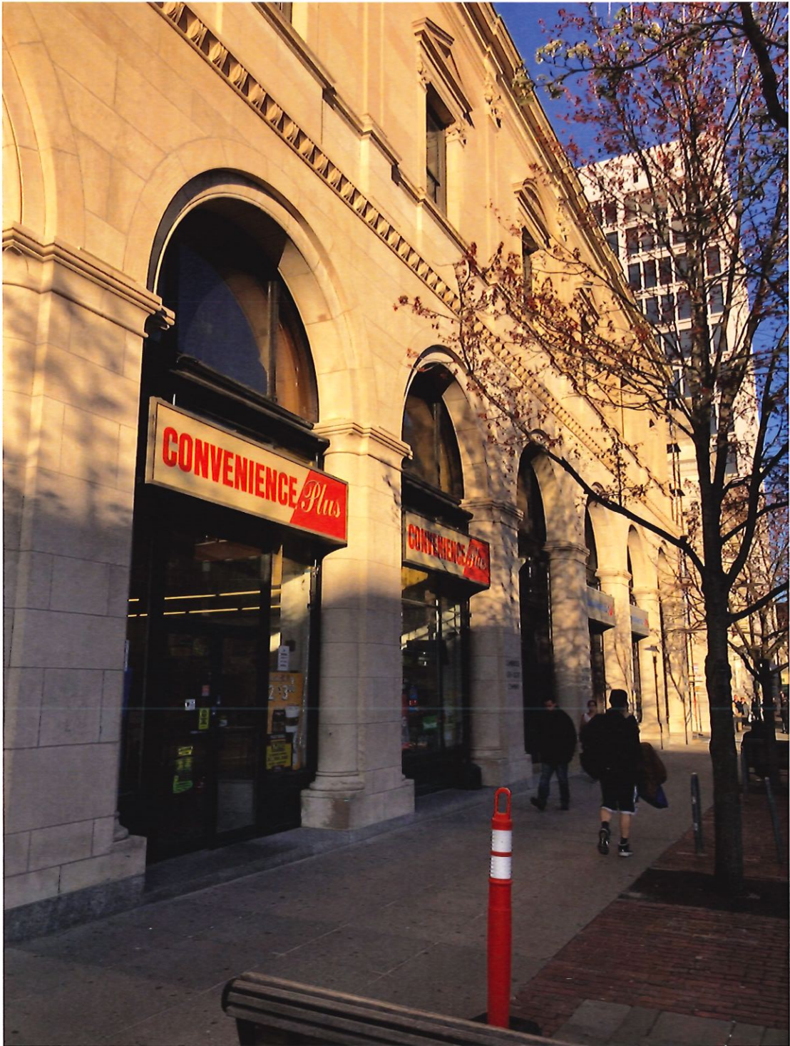
Closeup View from Massachusetts Ave Looking East
