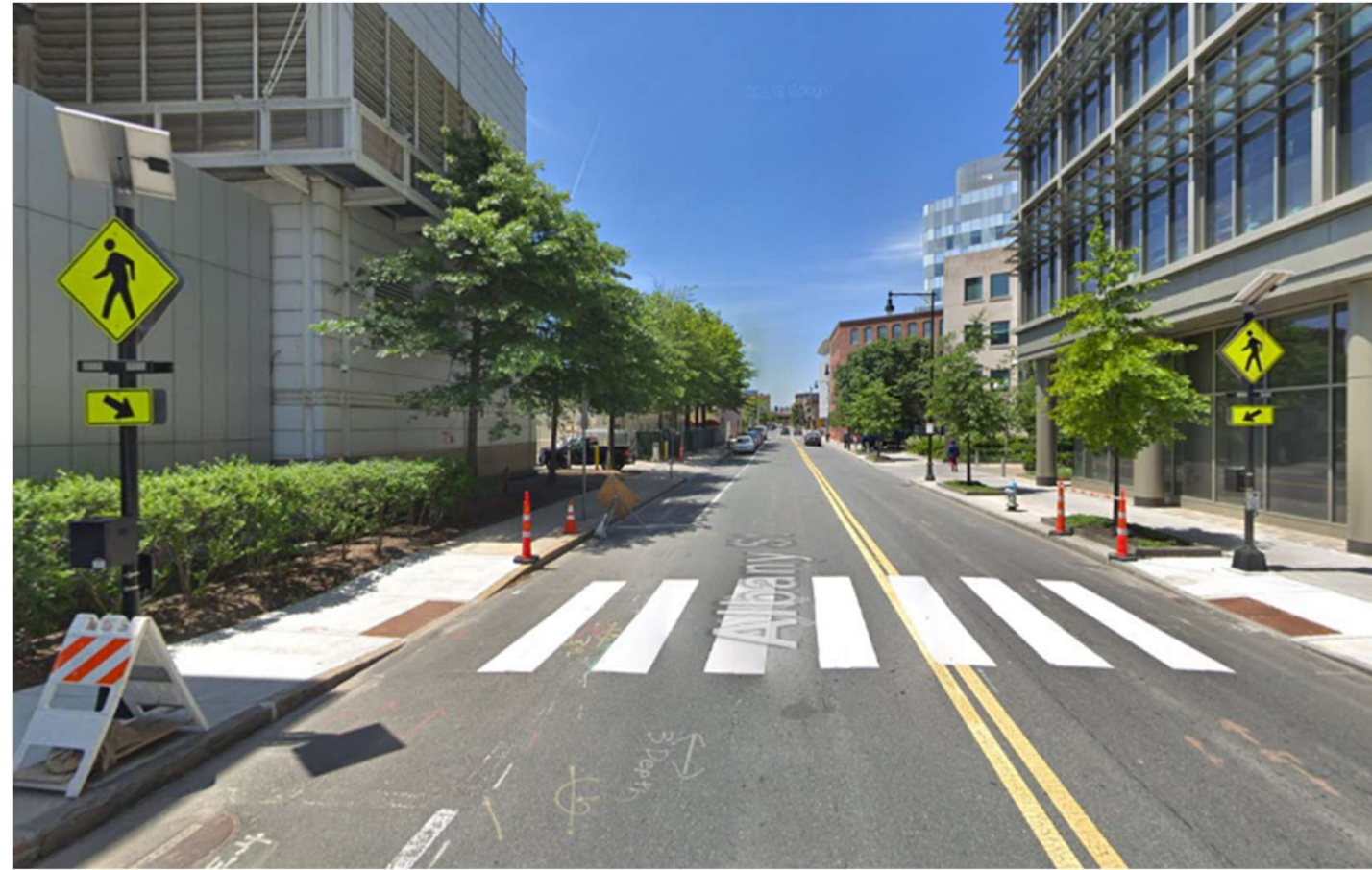
Photo: Example of RRFB on Albany Street at Portland Street
