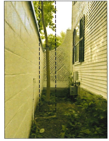
PHOTO #13 MISC-01: REMOVE TREE FROM GARAGE EAST FACADE.
