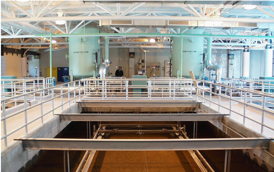
TYPICAL DAF INSTALLATION
