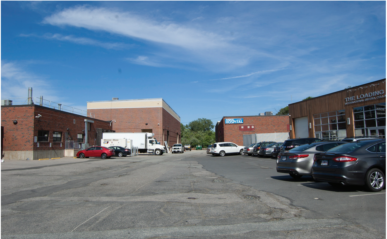
Single-story office and industrial buildings surrounded by parking exemplify the overall low building densities found in Alewife.
