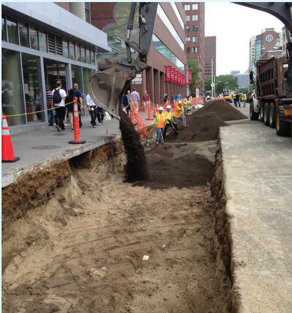
Main Street in Kendall Square showing the extent of sand based structural soil.
