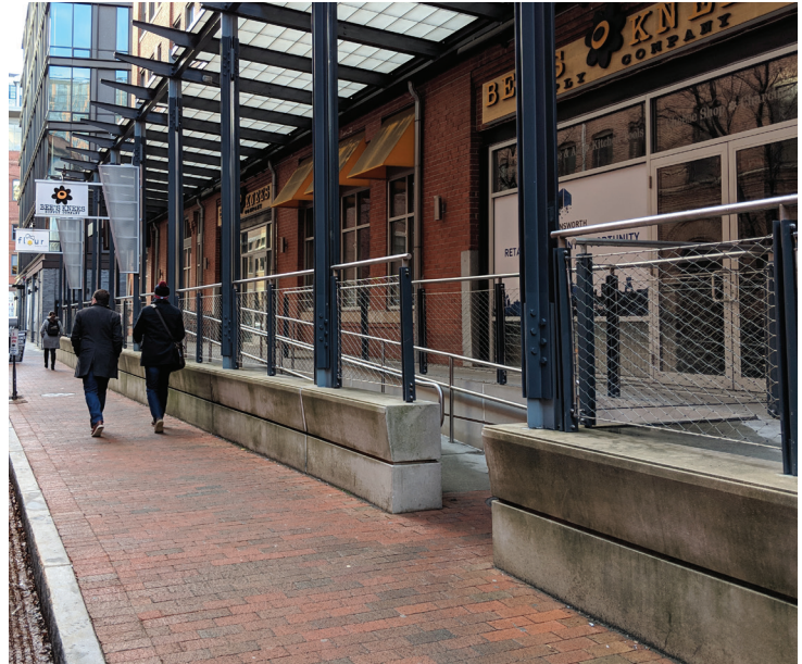
Elevated walkways are increasingly common today in potential flood zones, like Boston's Fort Point Neighborhood above.
