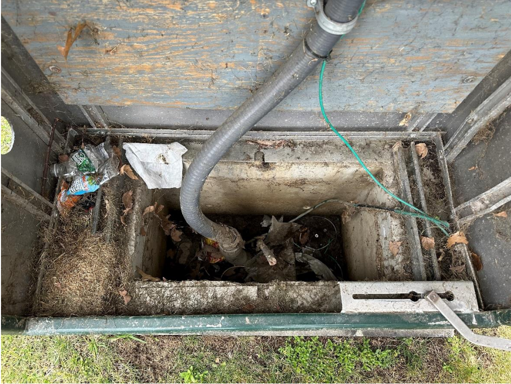
Electrical Cabinet Base
