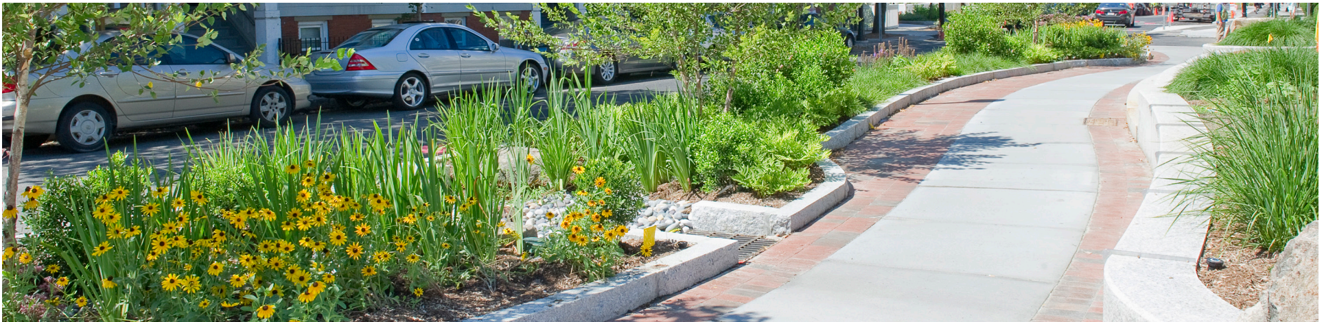
Figure 20. Integrating green infrastructure, like this rain garden, is a recommended early action for Stronger Infrastructure. Source: Kleinfelder
