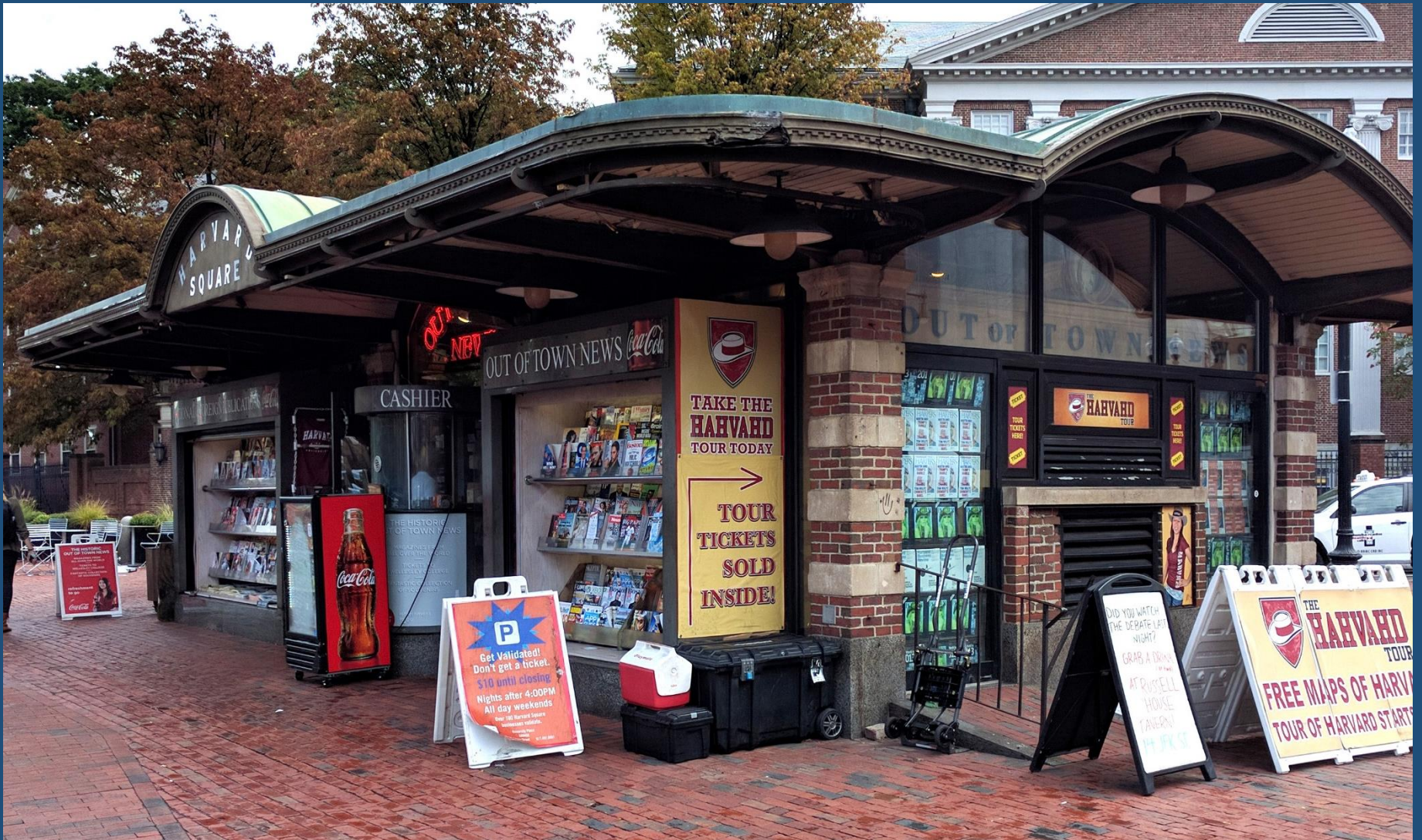
Harvard Square kiosk, west elevation, 2016 as remodeled in 1983
