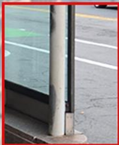
METAL TUBE AS COLUMNS
