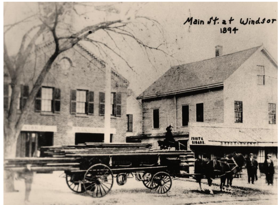
Image: Union No. 2 Engine House, 787-789 Main Street (at left), photo 1894. Courtesy Christian Mission Holiness Church, Cambridge Historical Commission
