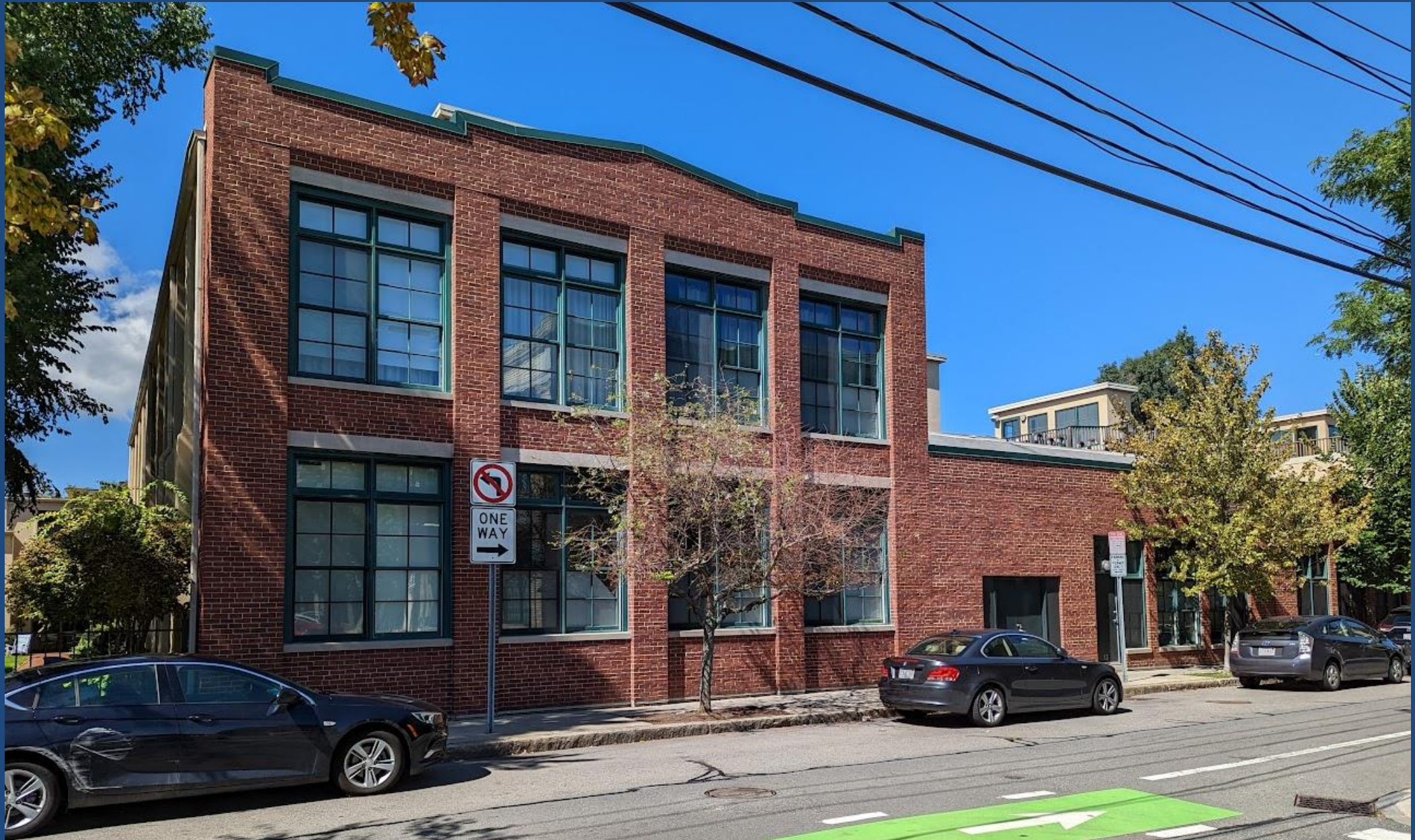
George H. Dyer Co. machine shop, 1914-1918. Converted to housing, 1997.
