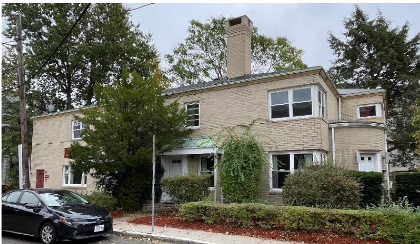
2161 Massachusetts Avenue, Milton Street elevation.
