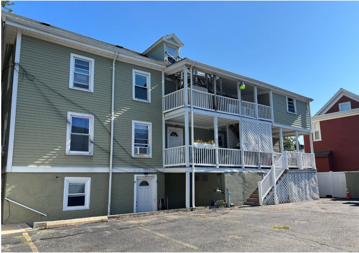
View of the rear of 42-46 Lincoln Street, CHC photo, 9/1/2023
