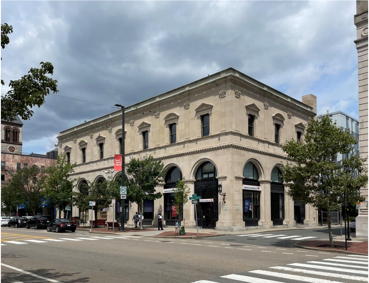
727 Massachusetts Avenue, Staff photo, 2021.
