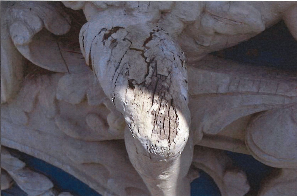
West cherub leg with end-grain exposed
