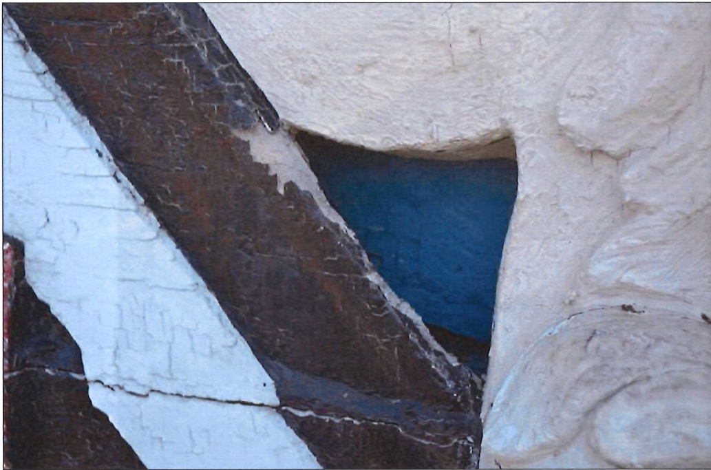
West showing horizontal cracks and location of seam from separate sections of carvings
