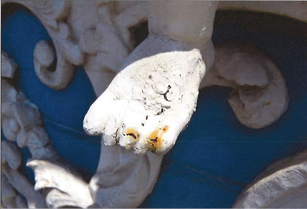
West cherub foot with ferrous metal fasteners at the toes
