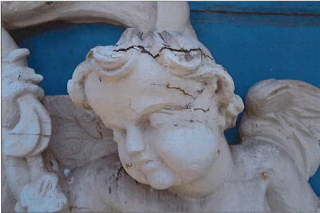
West cherub head with horizontal wood split
