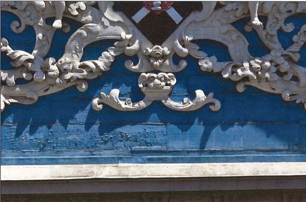
West wood dutchman repairs at backboards
