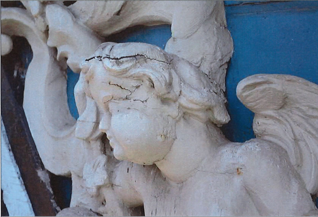
West cherub head with horizontal wood split
