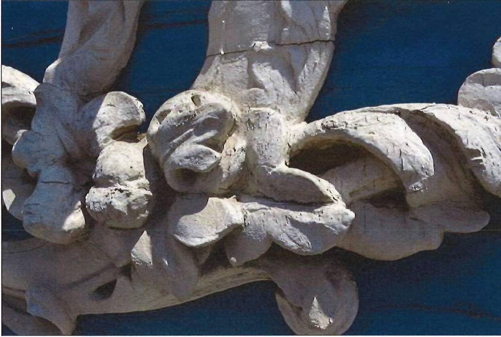
West showing horizontal cracks and location of seam from separate sections of carvings
