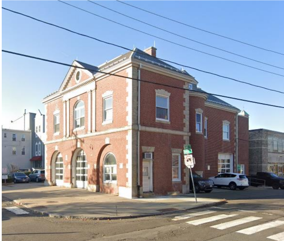
Example of Lightning Protection on City Electrical Shop located at 35 Third Street
