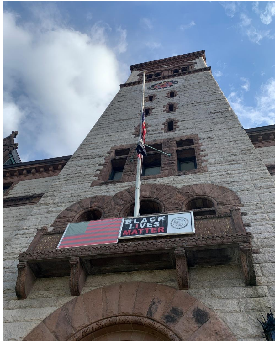
Existing Signage at Front of Balcony
