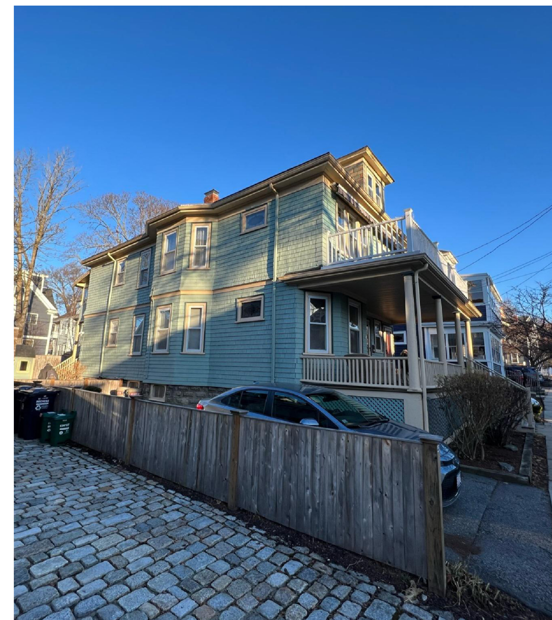
EXISTING WEST ELEVATION PHOTO
