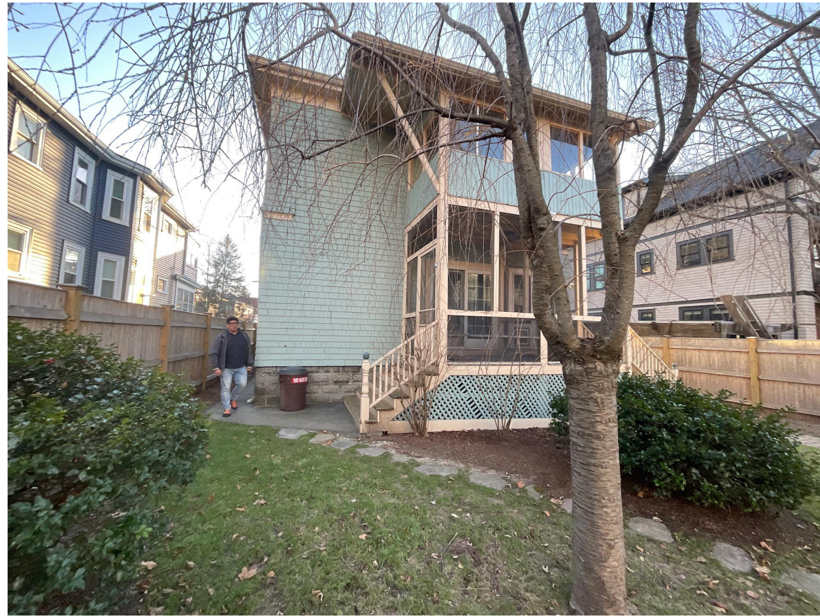
REAR PORCH & SIDE WALKWAY
