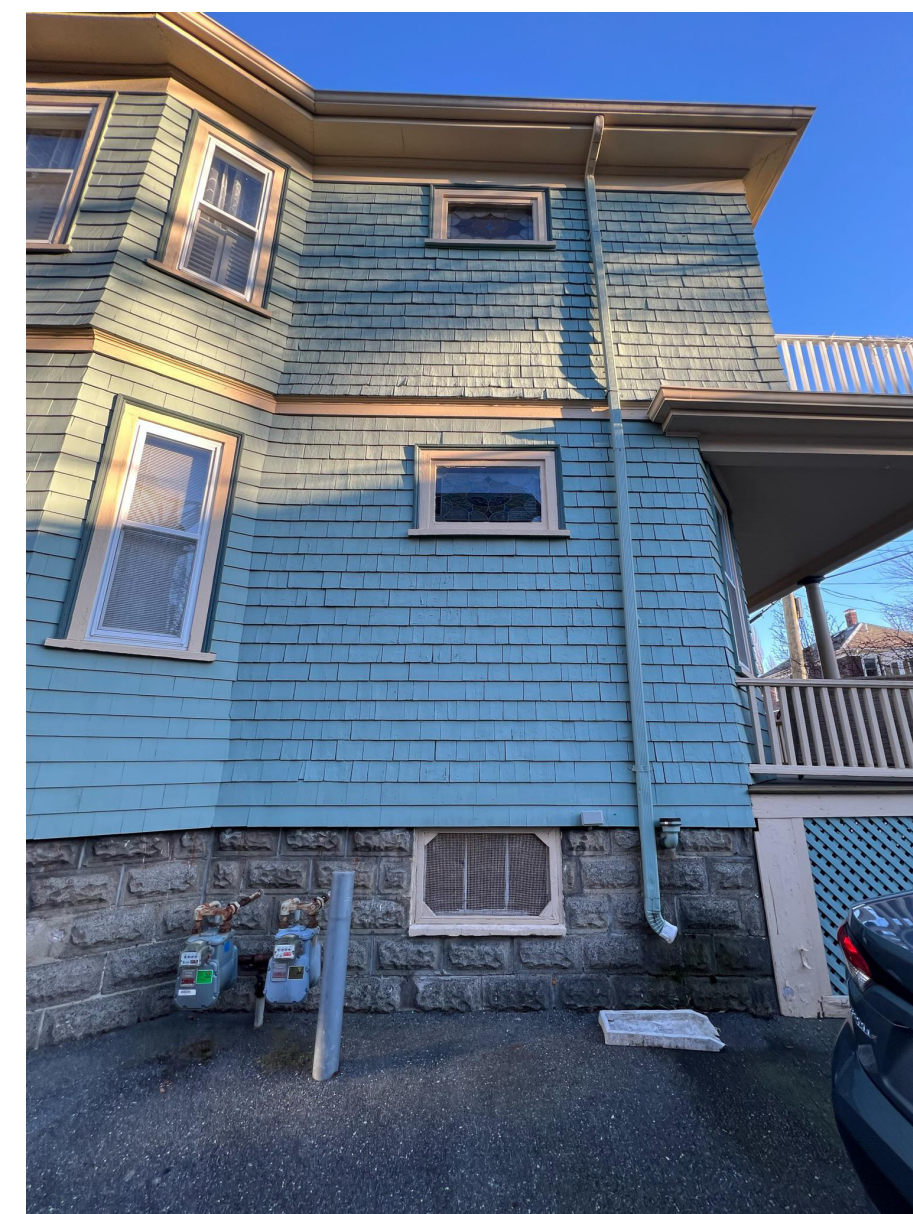
LEFT SIDE ELEVATION - DRIVEWAY & GAS METERS
