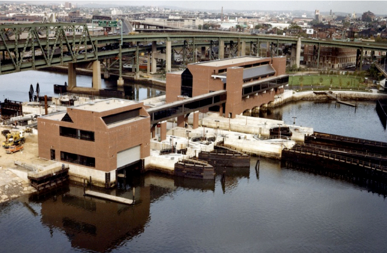
Charles River Dam (Source: New England District, US Army Corps of Engineers, 2015)
