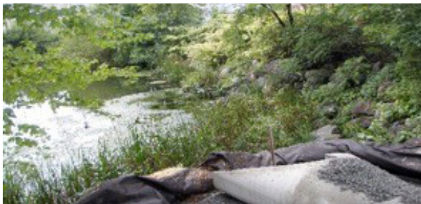
Figure 25. Retention Pond at the Waltham Polaroid redevelopment site [Source: Cambridge Water Department]
