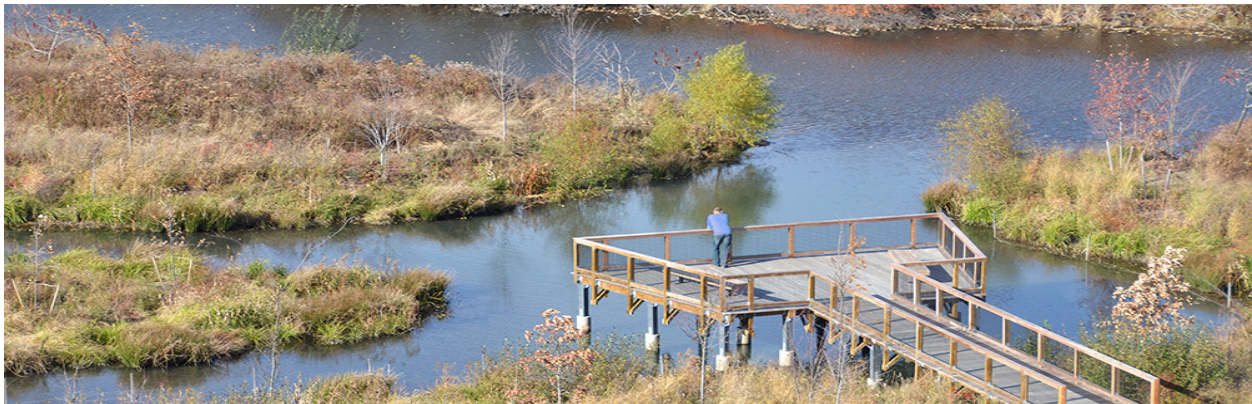
Figure 23. Alewife Constructed Stormwater Wetland [Kleinfelder, 2013]
