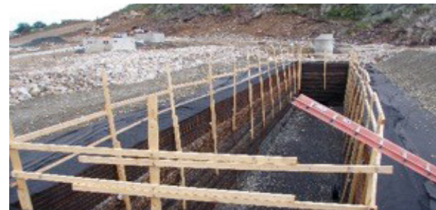
Figure 24. Underground infiltration basin under construction at the Waltham Polaroid redevelopment site [Source: Cambridge Water Department]
