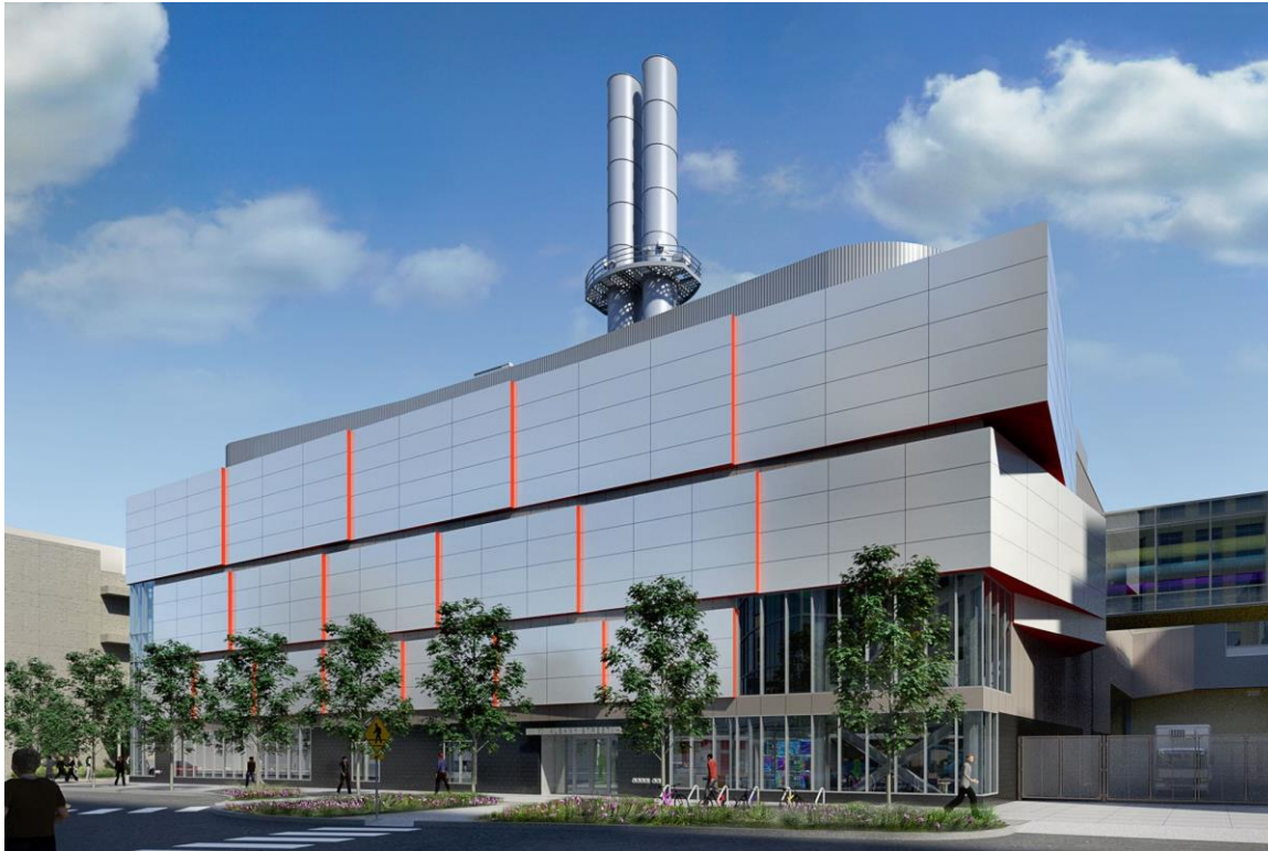
Conceptual sketch of the upgraded Central Utilities Plant at MIT, as viewed from Albany Street Credit: MIT/Ellenzweig.
