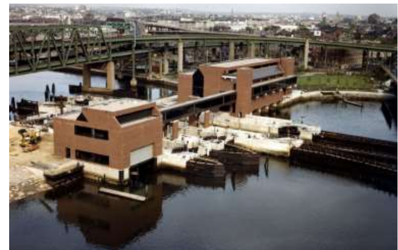
Charles River Dam (Source: New England District, US Army Corps of Engineers, 2015)
