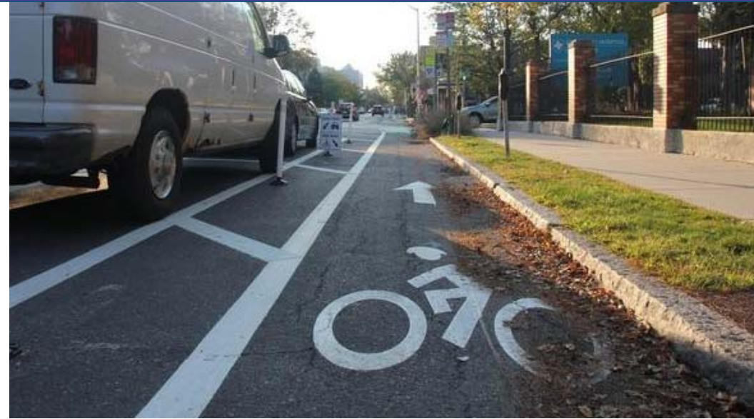
Example: Cambridge Street before the recent repaving
