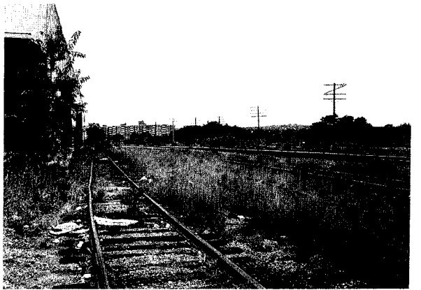
81. Underutilized Railroad Yards In the Alewife Industrial Area.
