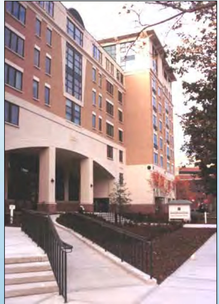
New residential development in the Triangle across from the T station
