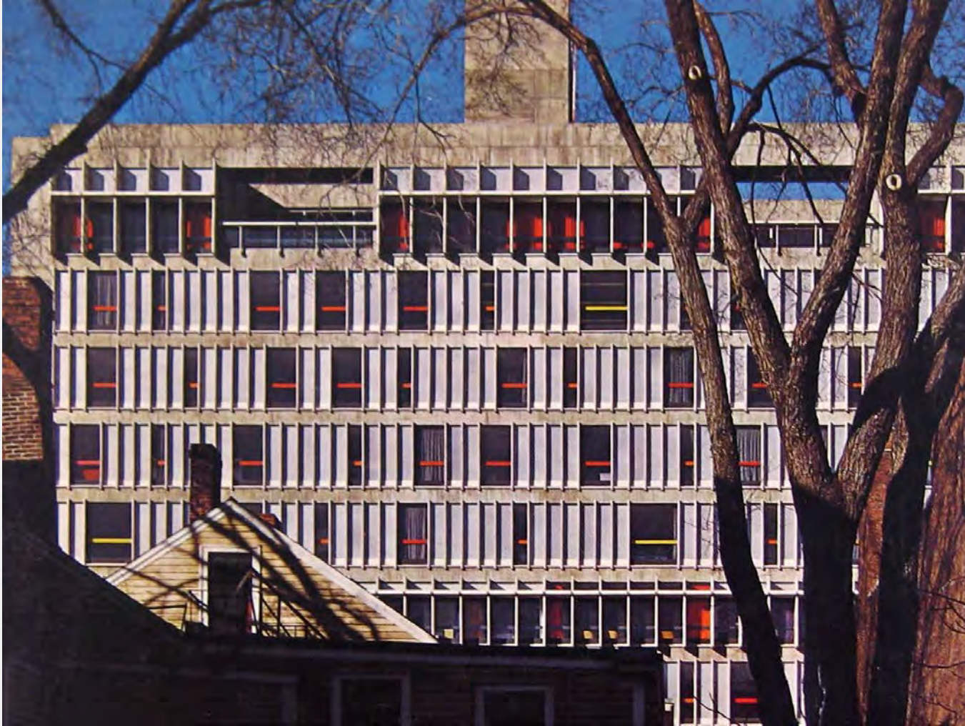
Building facade restoration • Bruner/Cott
