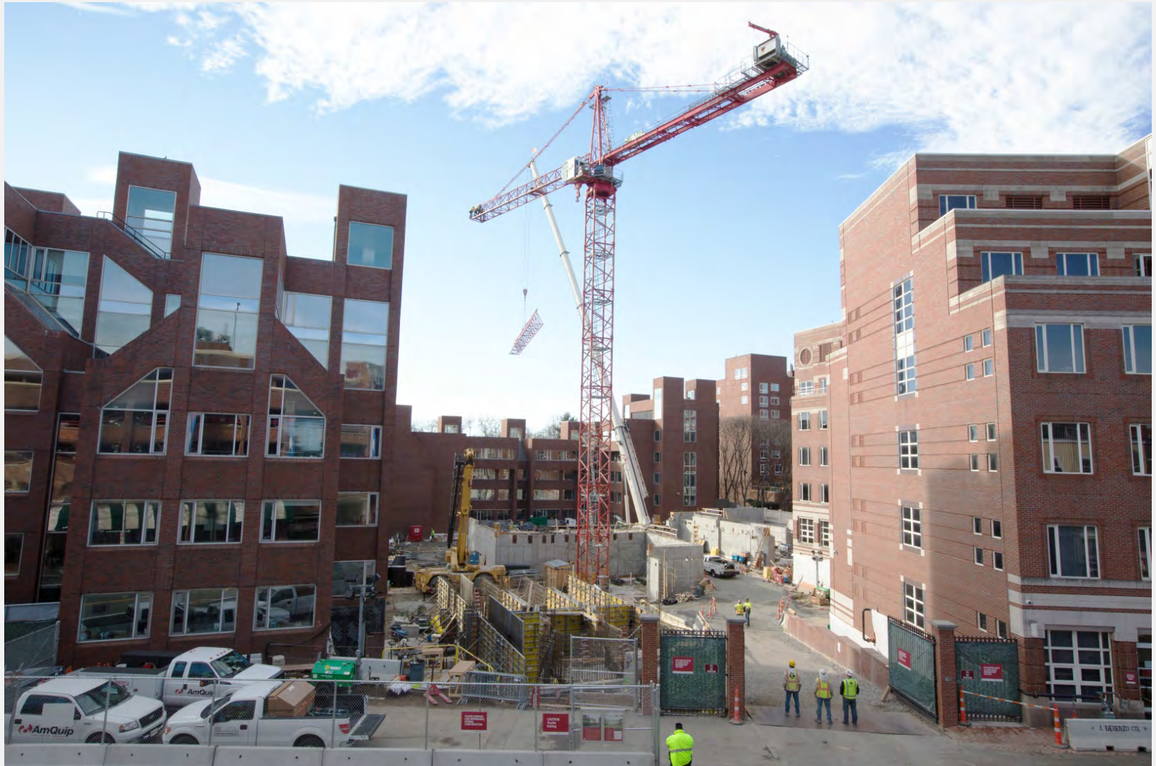
Construction of new academic space · Robert A.M. Stern Architects
