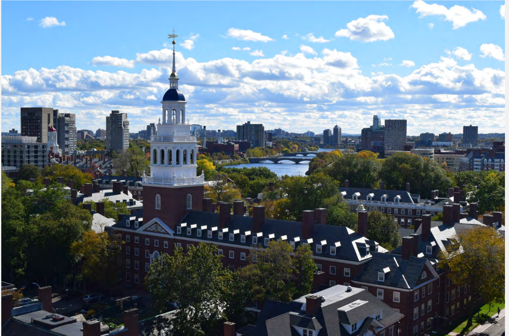
Comprehensive renewal of undergraduate House • Kieran Timberlake
