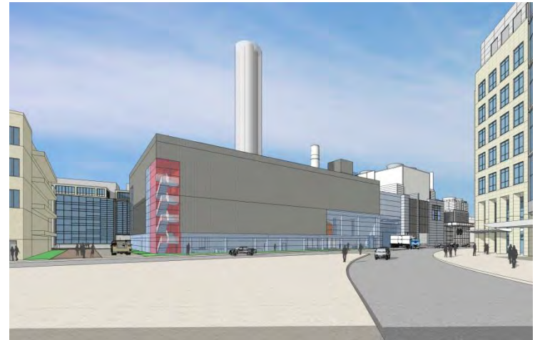
Central Utility Plant Upgrade
