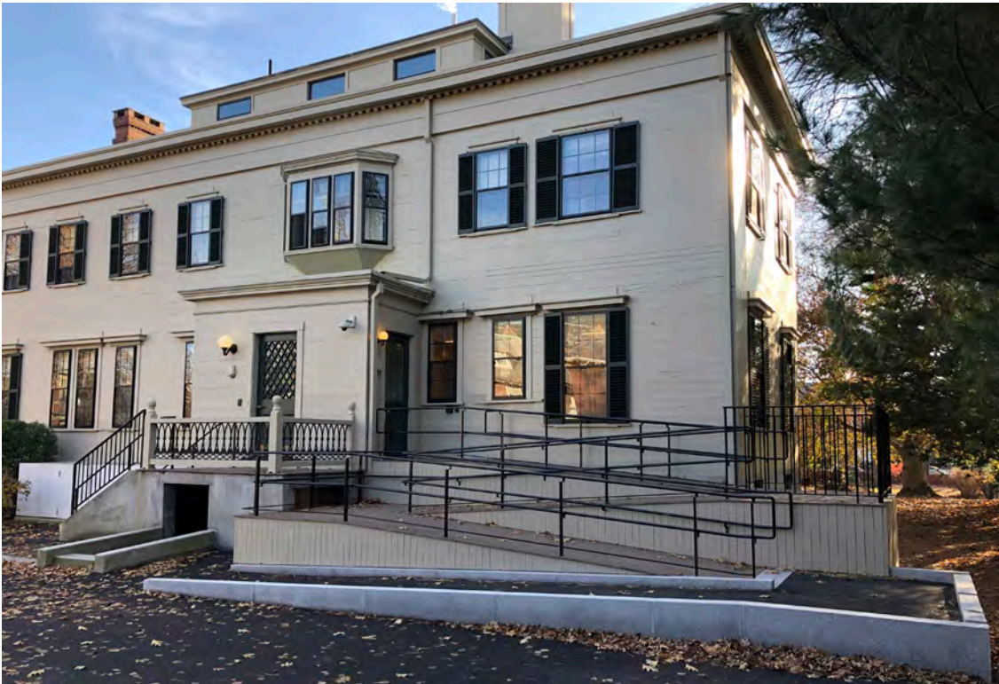
ONE OF FOUR RAMPS EITHER RENOVATED OR CREATED THIS PAST YEAR, THE RAMP TO 101 BRATTLE PROVIDES A GUARANTEED ACCESSIBLE ENTRANCE IN THE EVENT THE FRONT DOOR LIFT BREAKS DOWN.
