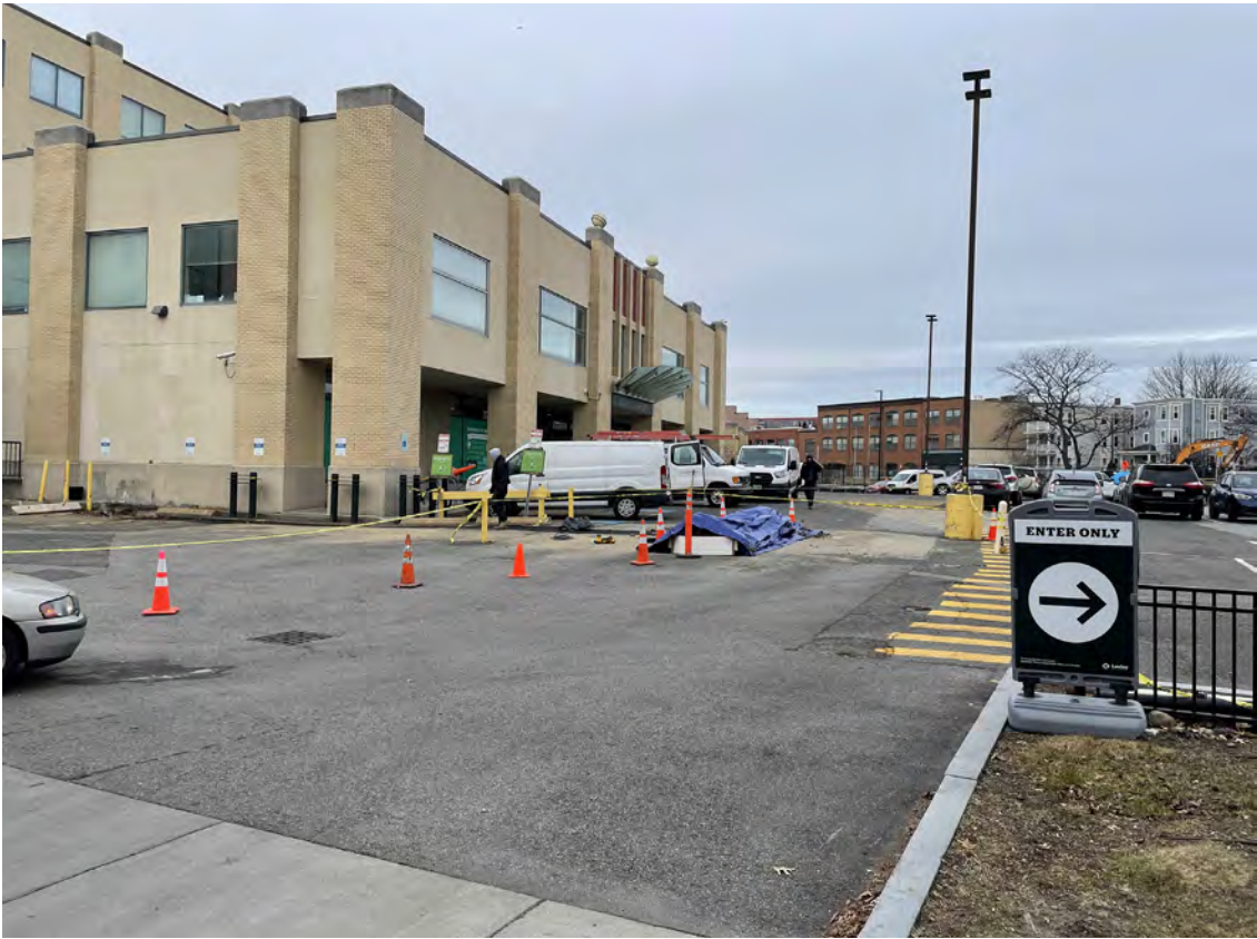
PARKING GATES AT UNIVERSITY HALL ARE BEING REPLACED WITH MODERN EQUIPMENT.
