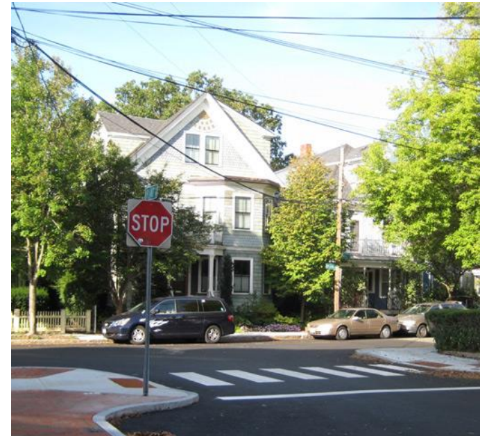
★ Curb Extension/Traffic Calming Program
