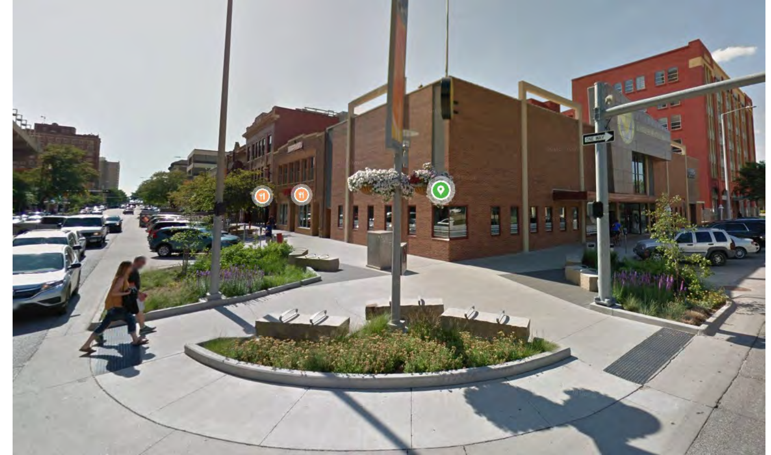
P STREET - LINCOLN, NE
