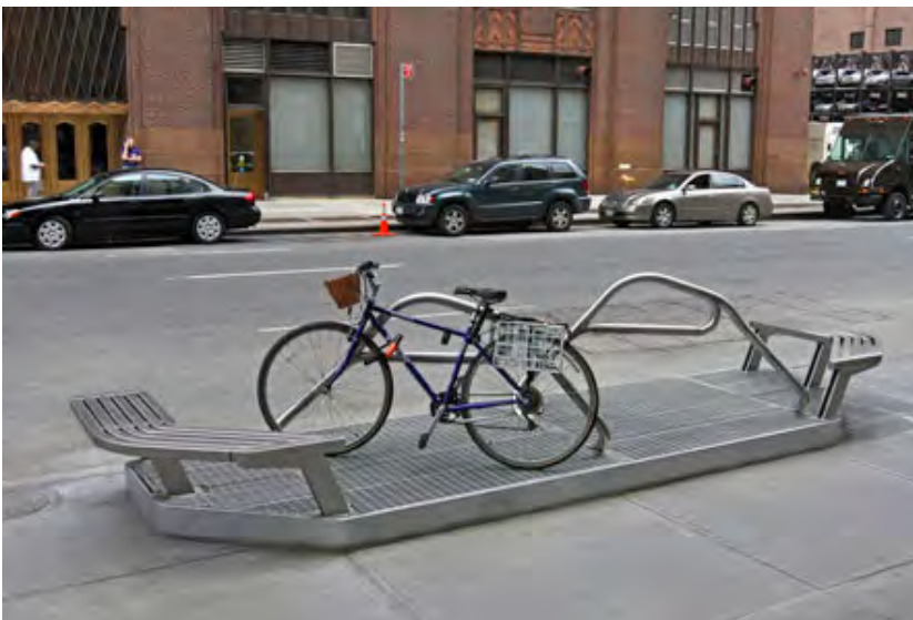
Figure 30. “Raised-grate street sculptures to prevent subway flooding. Stormwater improvements have been made at chronic flood locations by integrating raised-grate street sculptures to prevent subway flooding within the MTA NYCT service area and also serve as street furniture and/or bike racks.” Metropolitan Transportation Authority, New York City. 65
