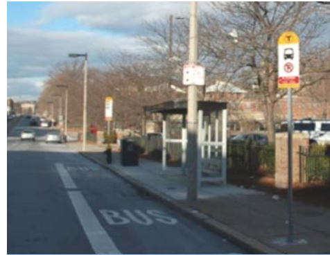
New Pavement Markings
