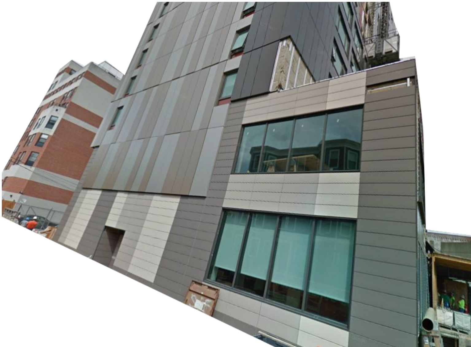
2. GREEN ST. - RESIDENTIAL Peter Quinn Architects LLC
