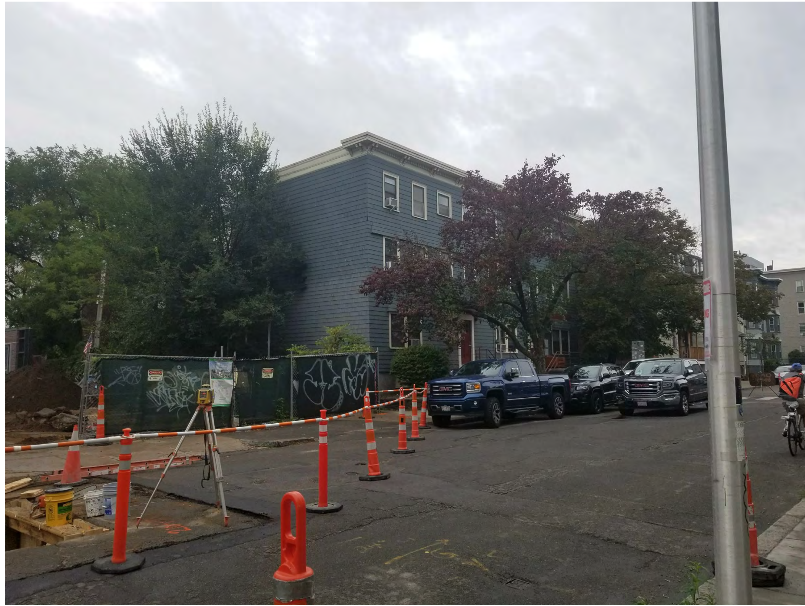
FRONT LEFT SIDE OF BUILDING (BISHOP ALLEN DRIVE)
