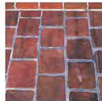
Quarry tile to terraces : relaid
