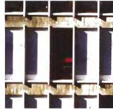
Cast in place slab edges
