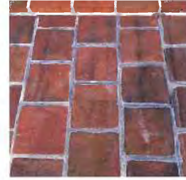
Quarry tile to terraces
