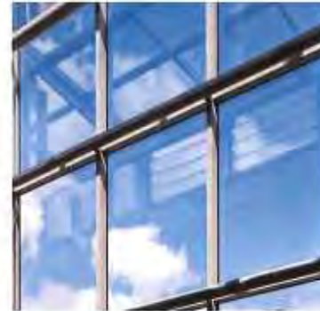
Metal framed glazing
