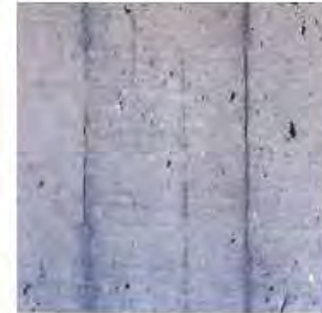
Cast in place concrete cleaned
