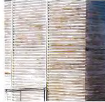
Painted metal louvres
