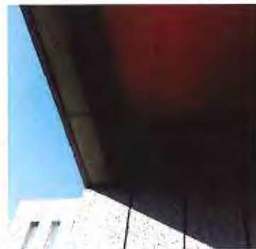
Painted concrete soffits
