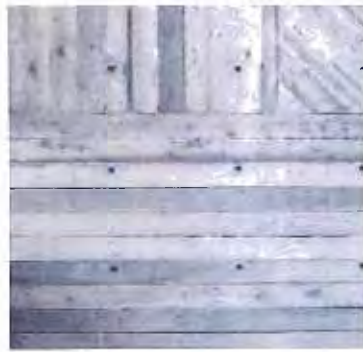
Cast in place
