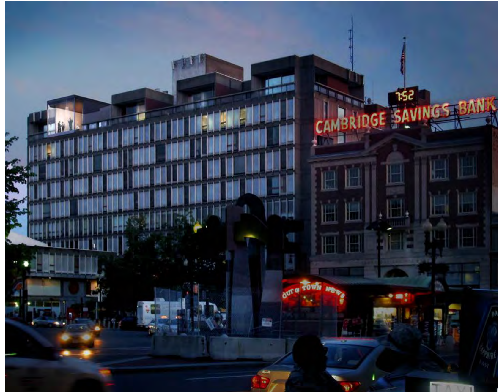
View from Massachusetts Avenue showing new "beacon" at the roofline of the building
