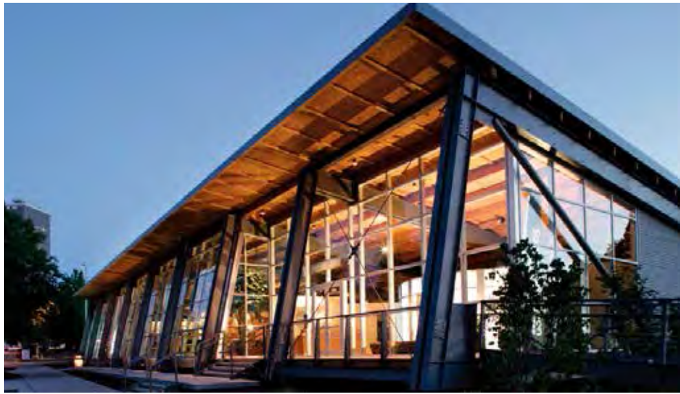
Framed glass facade: Pavilion Park, Seattle WA
