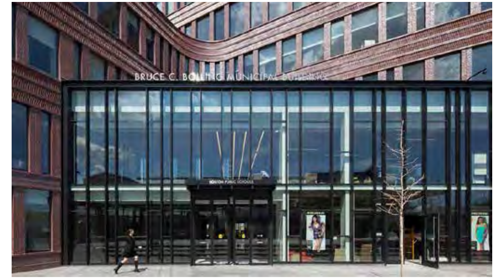
Framed glass facade engages public: Municipal Building, Roxbury MA
